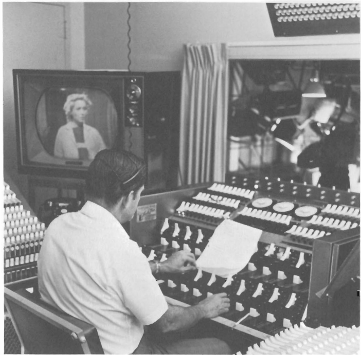
Television's technical capabilities were vastly expanded recently in conversion to almost complete color broadcasting. Above is latest in studio lighting control—hundreds of switches providing director with almost limitless variety and flexibility in lighting.
